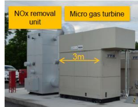
NH 3 -kerosene-air micro gas turbine in our institute (AIST)
