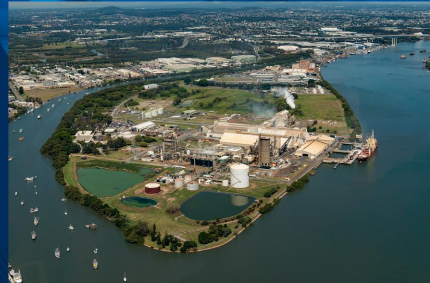
IPL Plant in Brisbane, Australia
