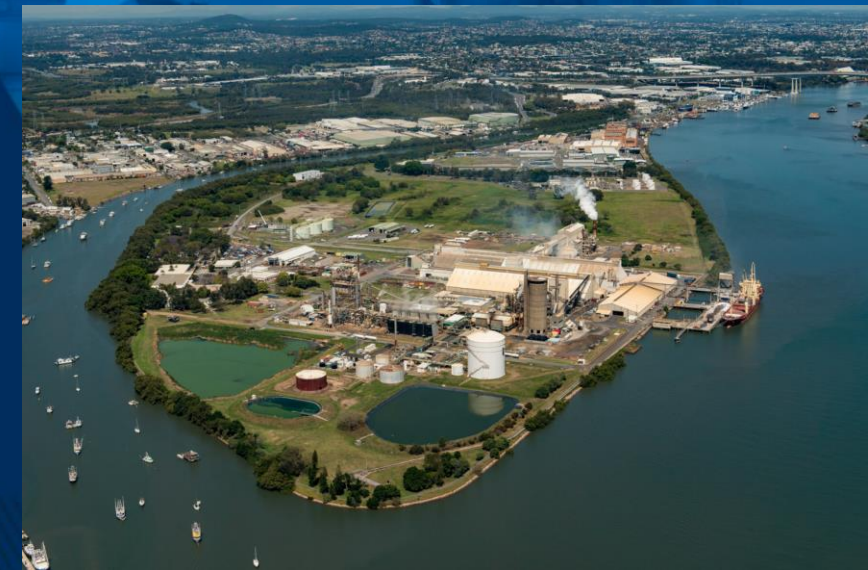
IPL Plant in Brisbane, Australia
