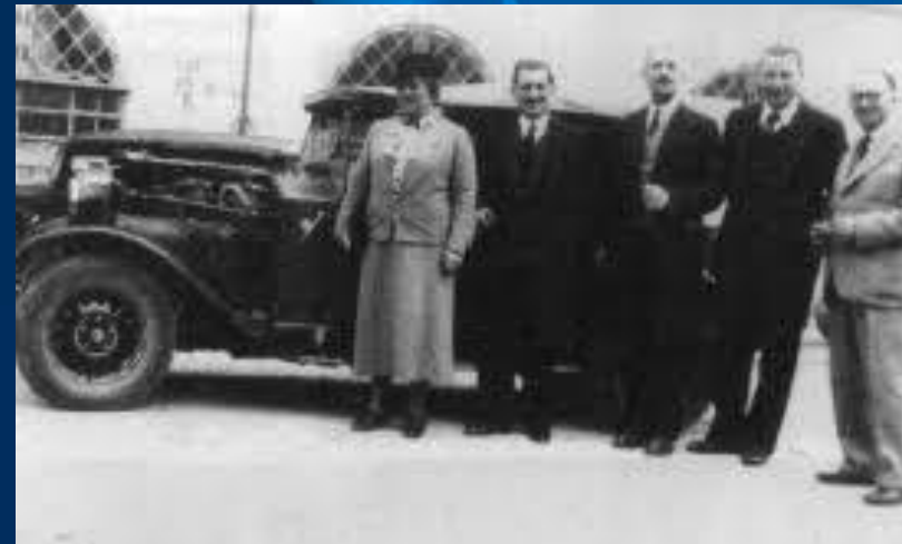
Fiat car with engine fuelled with ammonia. Casale patent in 1935
