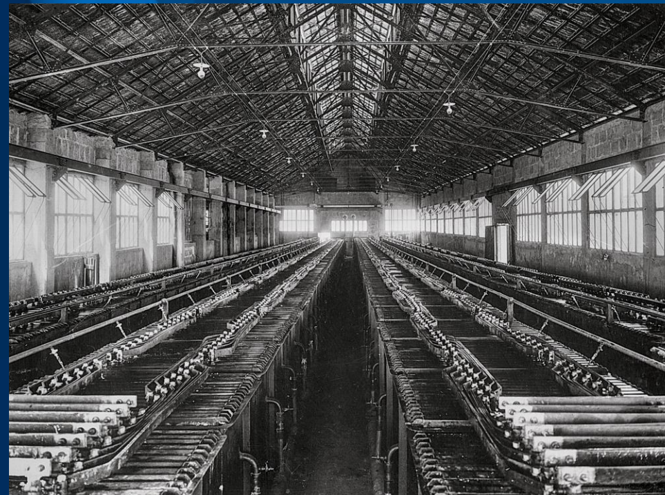
Casale Water Electrolyzers
