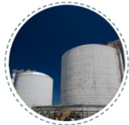
3 Ammonia Tank 100k Ton
