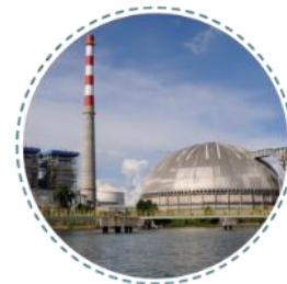
Coal Boiler 560 Ton per Hours
