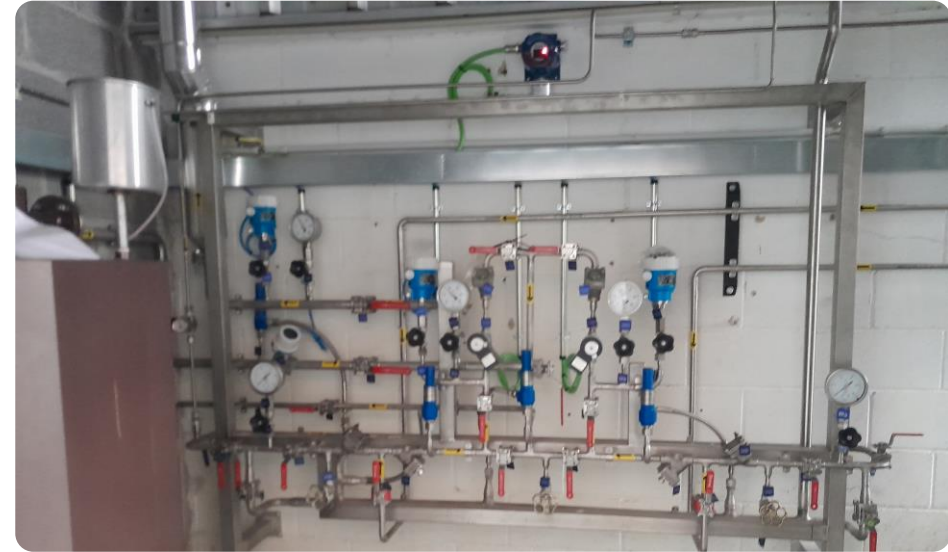
Safety logistics handled in installation phase
