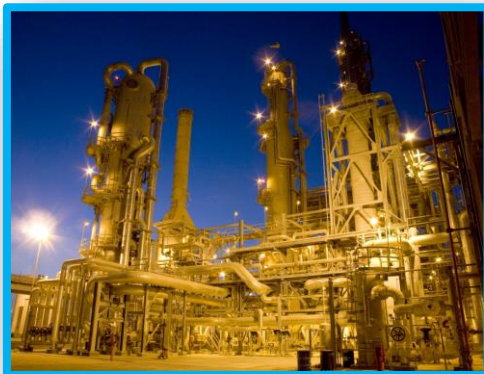
ammonia: zero-carbon fertiliser, fuel and energy store
