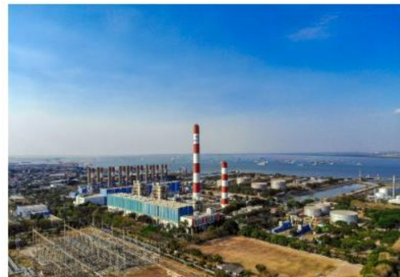
PNP's Gresik Thermal Power Plant
