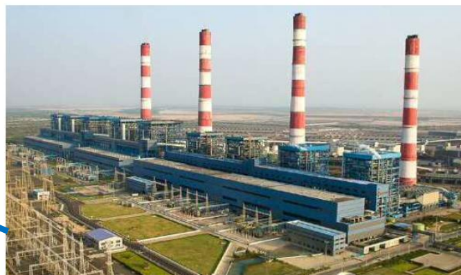
Mundra Power Plant
