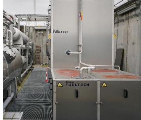
Ammonia supply and recirculation system
