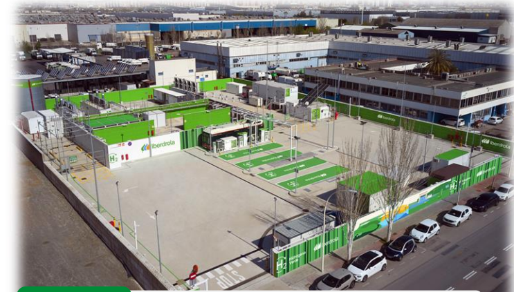
2.5 MW H2 station in Barcelona
