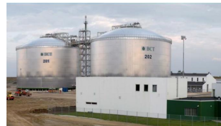
40,000T tanks for anhydrous ammonia, Netherland
